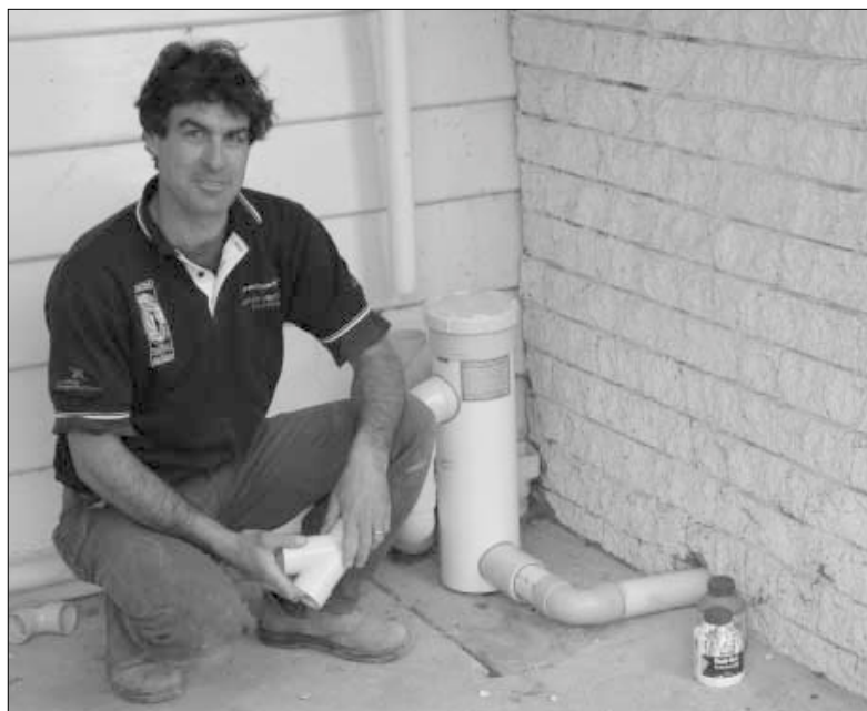
The Greywater Saver is a diversion and filtration greywater system.
